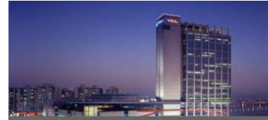
Gangbyeon Techno Mart
